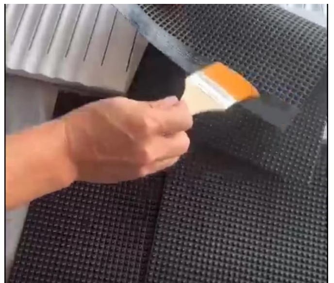
4-Repeat the previous process on the smooth edge of the side strip of the mat from the front side, using a brush along the length of the mat roll with an area of 2-3 cm
